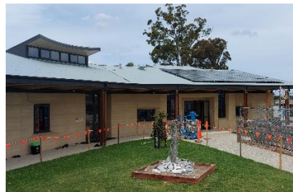
The new Clifton Creek Primary School, now completely rebuilt with a REC Alpha system
