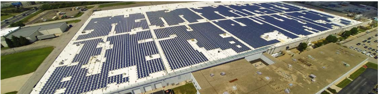
Rockville Solar II - 3.2MW - 4.3million kWh/year - 12,264 REC solar panels - Indianapolis, Indiana - by Melink Corp.
