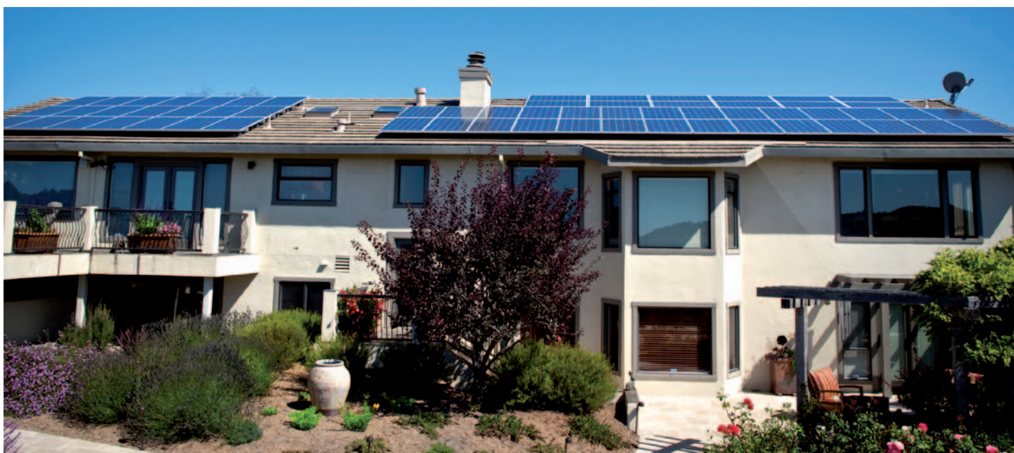
Evans Family Home - 13.4 kW - 19,435 kWh/year - 19,526 REC solar panels - Monterey, California - by REC Solar Inc.
