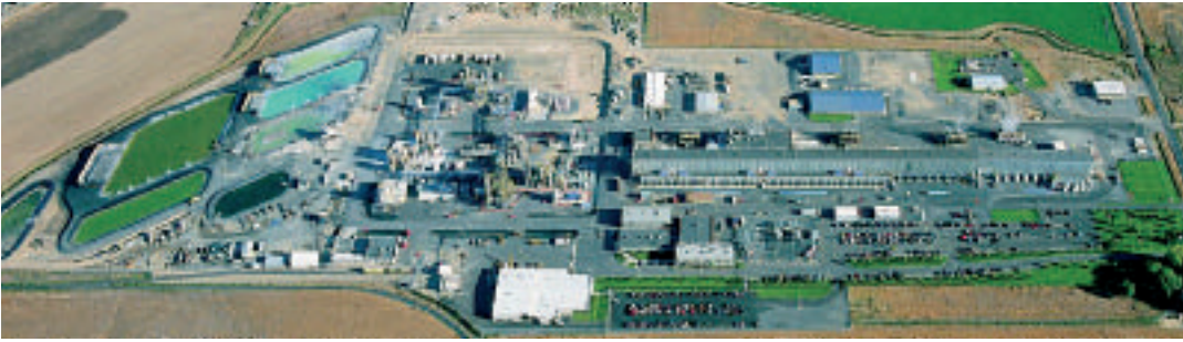
Overview of the SGS plant in Moses Lake, Washington, USA.
